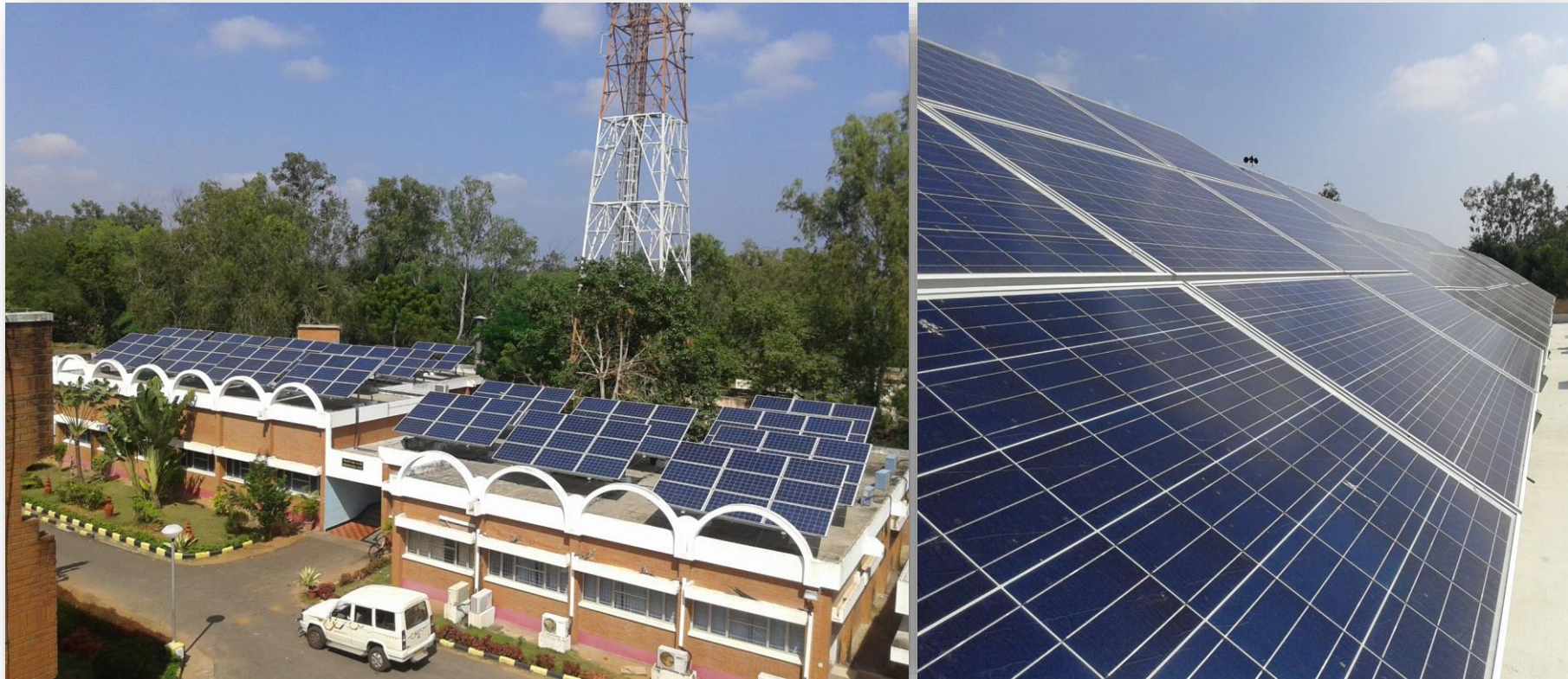
ISRO - 3060 KW SOLAR ROOFTOP INSTALLATION
